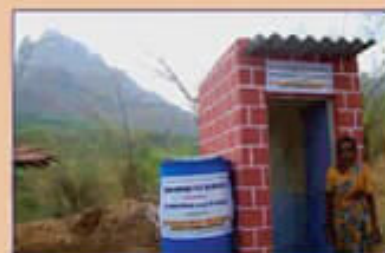
Toilet Block Project
